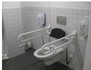
Blick in das WC
